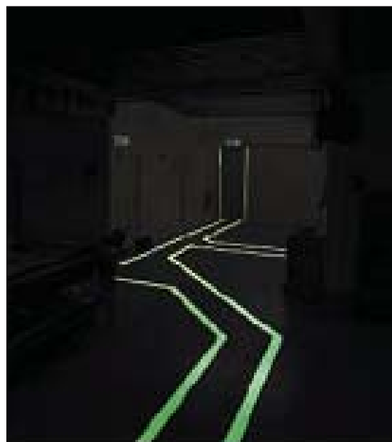
Figure 48: A 'way-guidance' system
