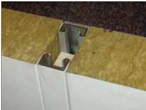
Figure 16: Insulated core panels – internal panel
