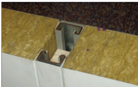
Figure 17: Insulated core panels – internal panel
