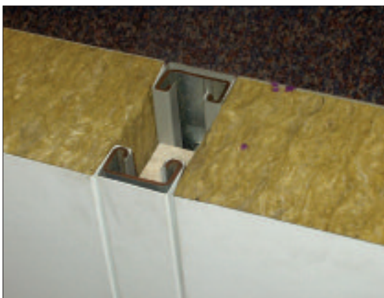
Figure 17: Insulated core panels – internal panel
