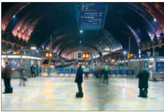
Figure 30: A covered railway station
